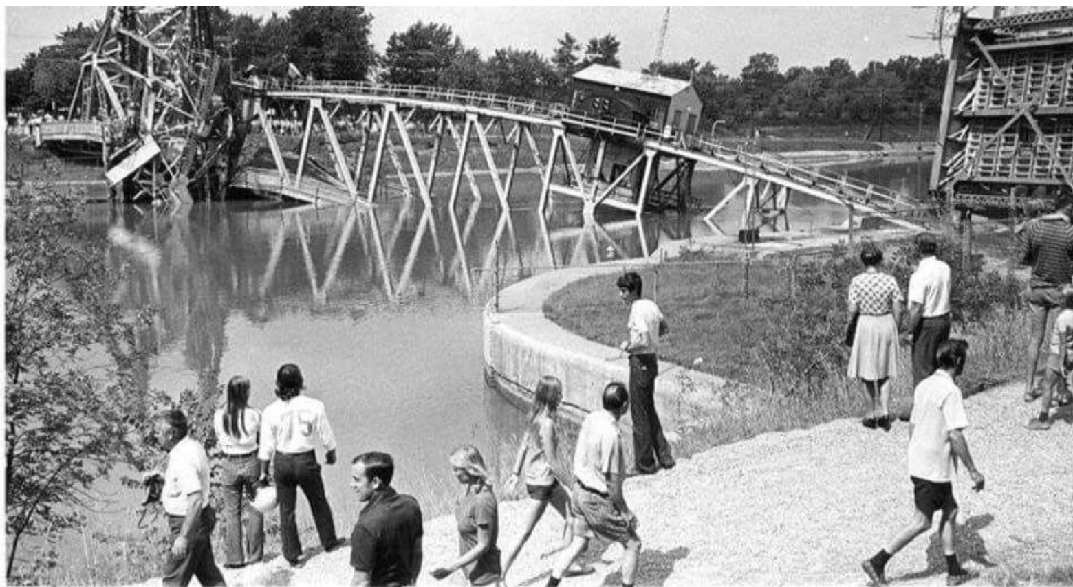
PORT ROBINSON BRIDGE - AUGUST 25, 1974
