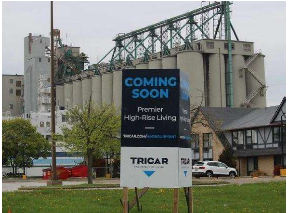
A sign advertises a high-rise development proposed near the Cargill grain terminal on Sarnia Harbour. Photo by Paul Morden /The Observer
