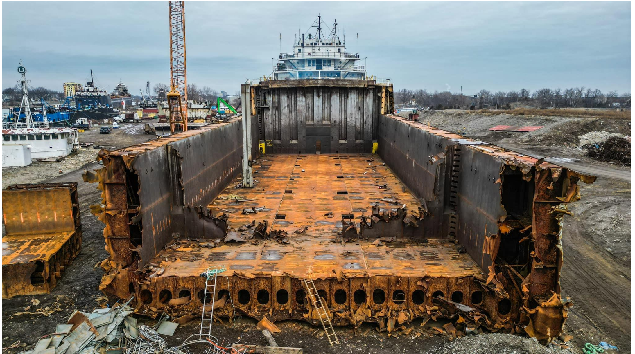
A look at the structural makeup of the cargo hold.
