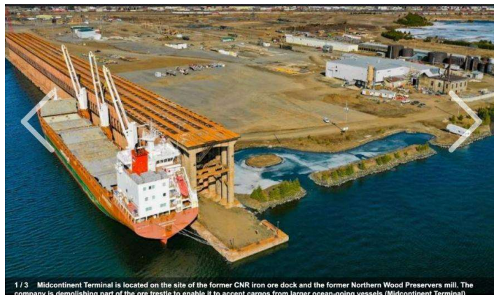
1 / 3 Midcontinent Terminal is located on the site of the former CNR iron ore dock and the former Northern Wood Preservers mill. The company is demolishing part of the ore trestle to enable it to accept cargos from larger ocean-going vessels (Midcontinent Terminal)
