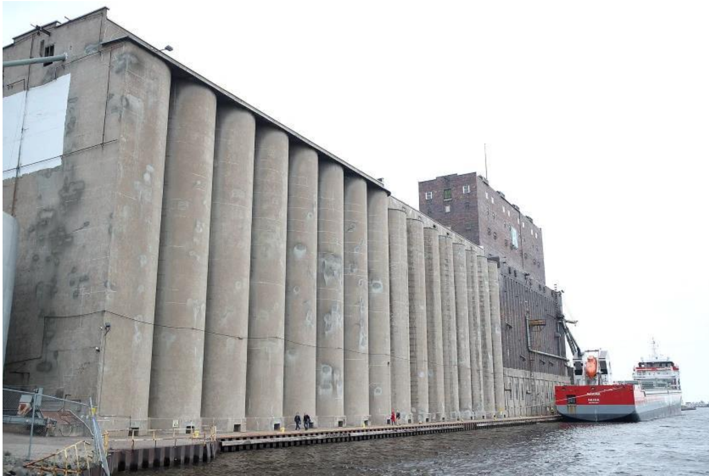
Duluth's Elevator A sees first ship in nearly a decade
