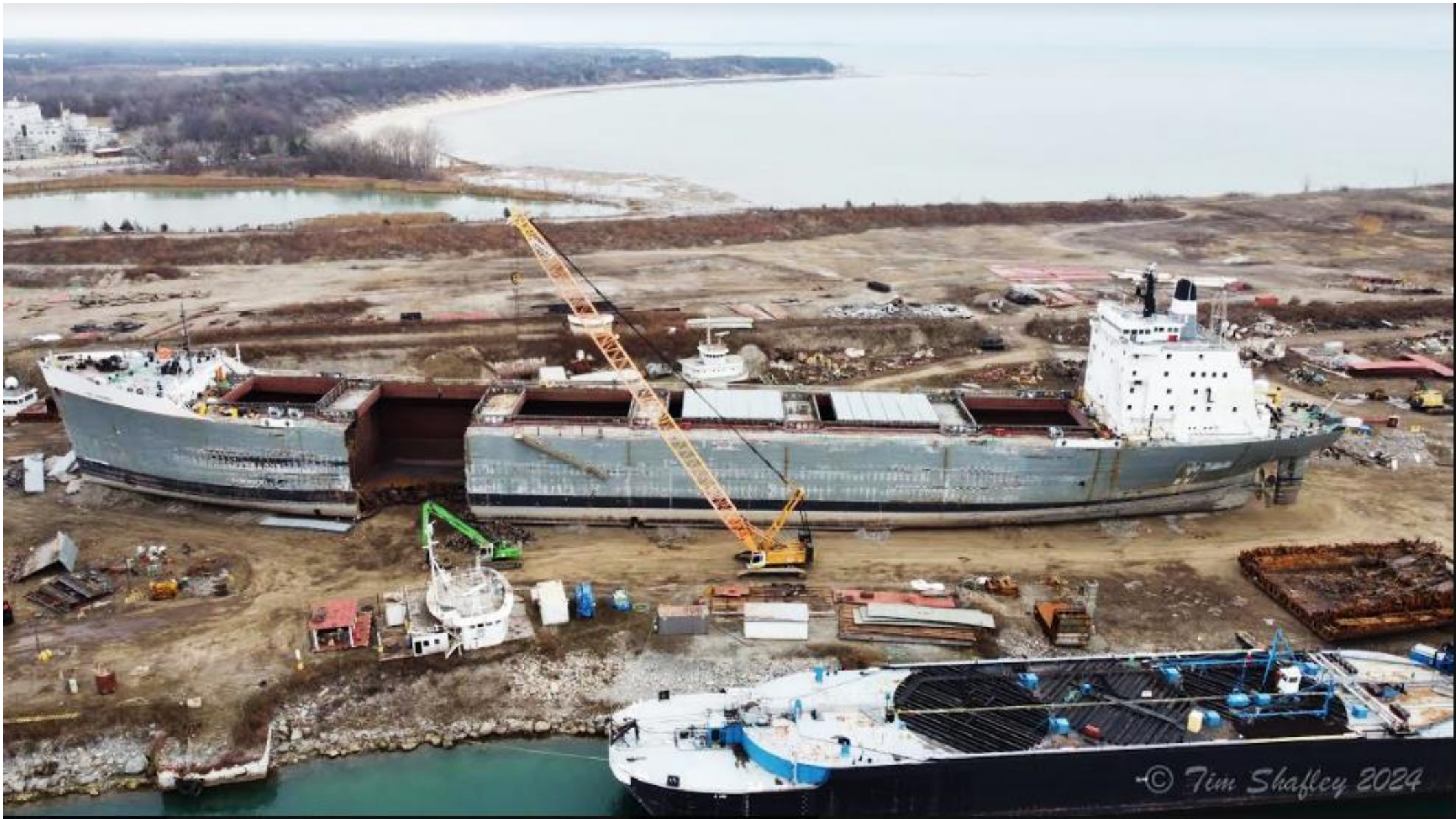
Scrapping well underway on the Tecumseh [Tim Shafley]
